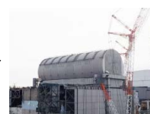
Completion of cover structure
