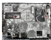
After Rubble Removal
