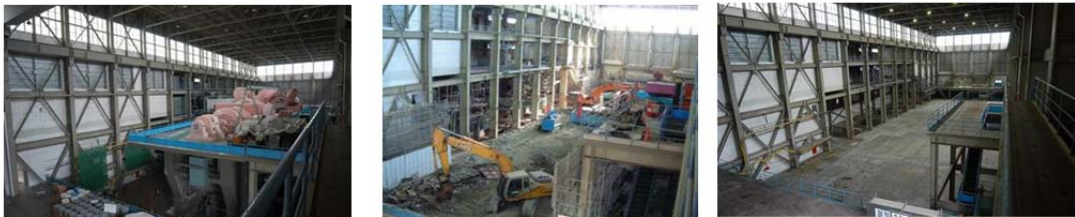
Removing work of the Turbine and Generator at Tokai nuclear plant
