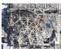
Before Rubble Removal
