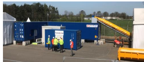
Figure 1. On-site installation of FREMES
