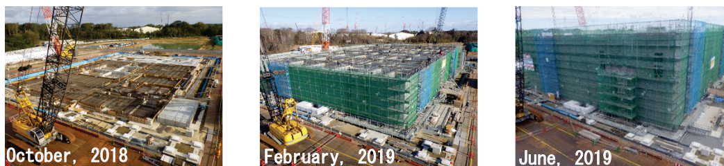
Fig. 2: Construction status of Laboratory-1
