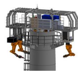
Cutting of Stack Shaft
