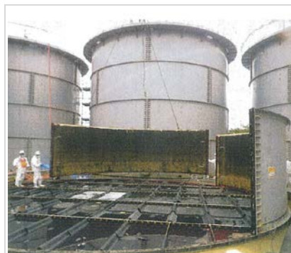
Figure-1 Dismantling flange tank status
