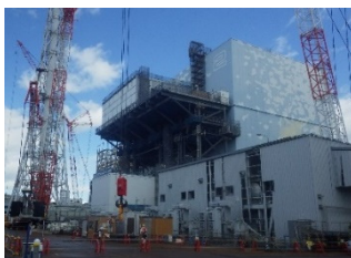
West platform construction
