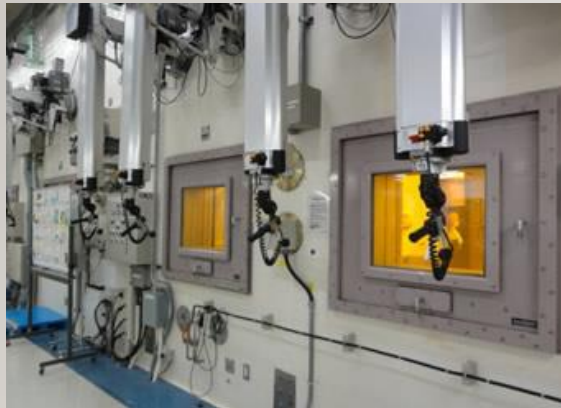
Concrete Cell with manipulators
