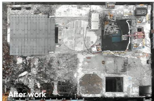
Removal of scattered debris on top of Unit 3
