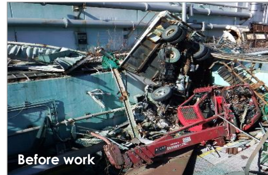
Removal of tsunami debris
