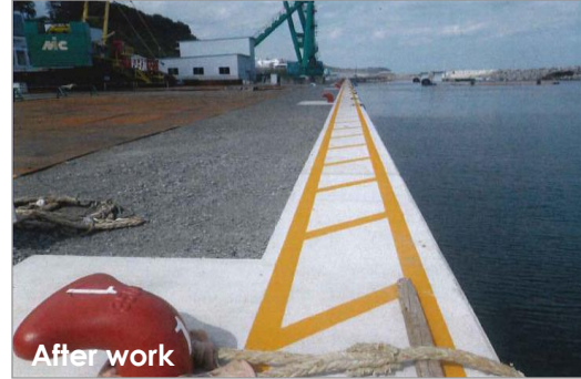
Restoration of revetment at shallow draft quay
