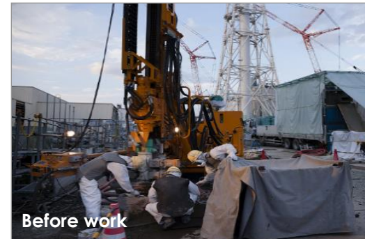
Installation of land-side (frozen soil) impermeable wall
