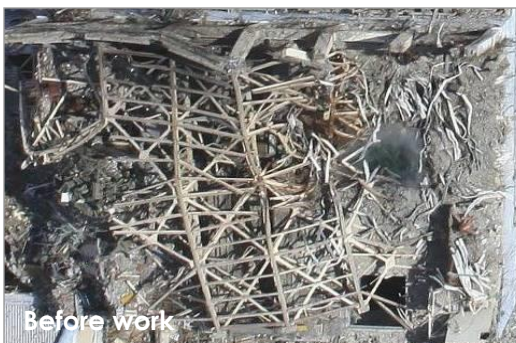
Removal of scattered debris on top of Unit 3
