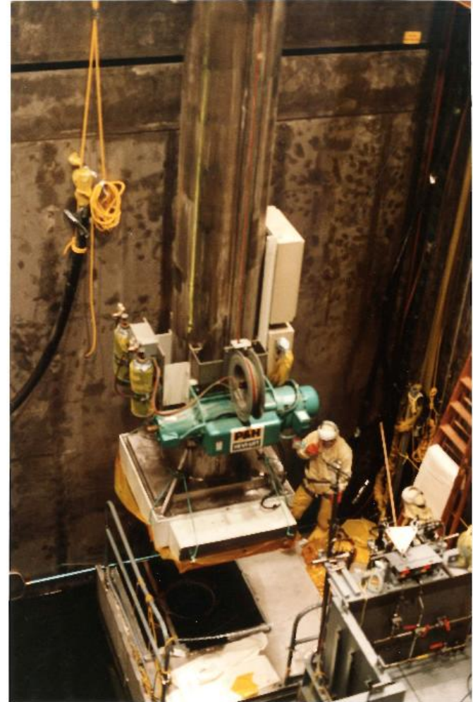
Transfer Cask Operations
