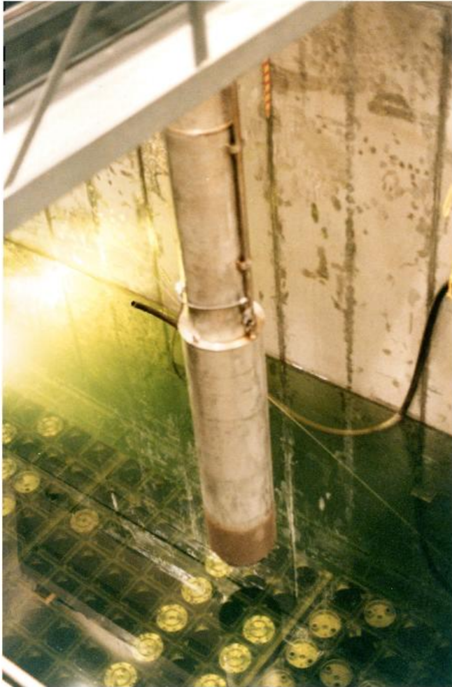
Canister Staging in Spent Fuel Pool
