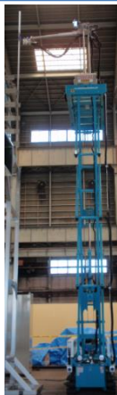
Dry ice blast
