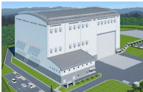
JAEA, Naraha Remote Technology Development Center Test building
