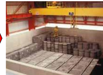
Surface disposal for IL-SL waste
