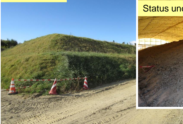
Soil covered temporary storage facility (30mSv/h or less, plus rubbles from 1 to 4 reactor building)
