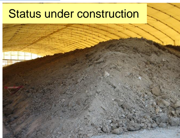
Soil covered temporary storage facility (30mSv/h or less, plus rubbles from 1 to 4 reactor building)
