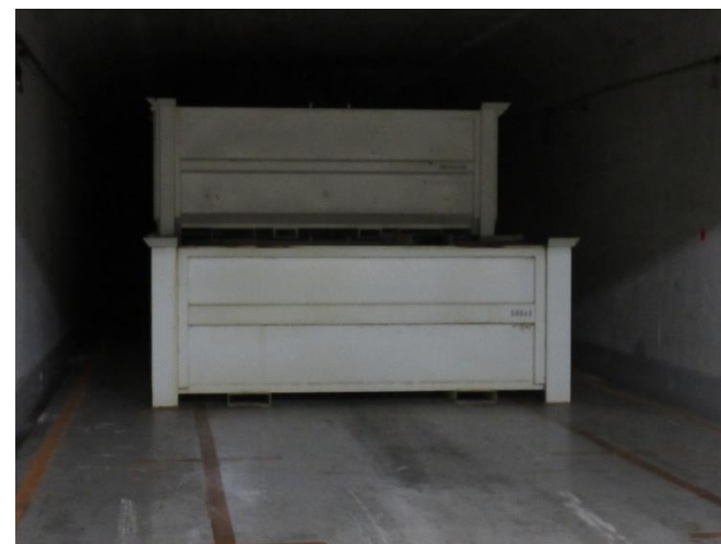
Solid waste storage building (More than 30mSv/h)
