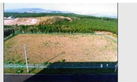
Overview of the Disposal Facility Covered with Soil (1997)
