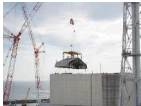
Removal of last one roof panel
