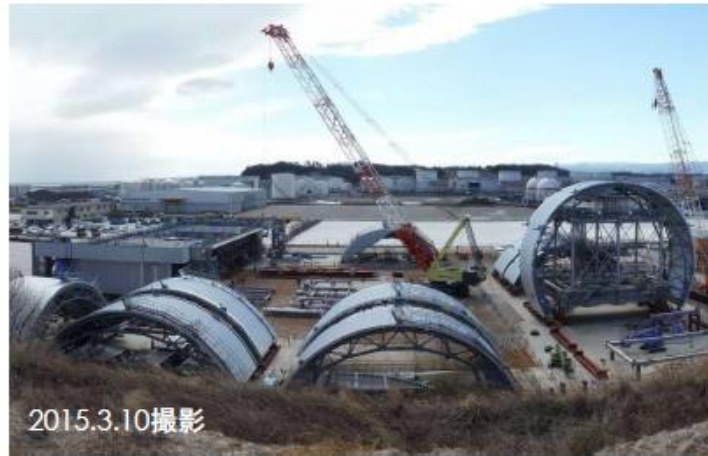
Building covers under fabrication
