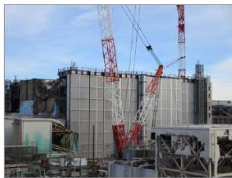
During preparation of retrieval/decontamination
