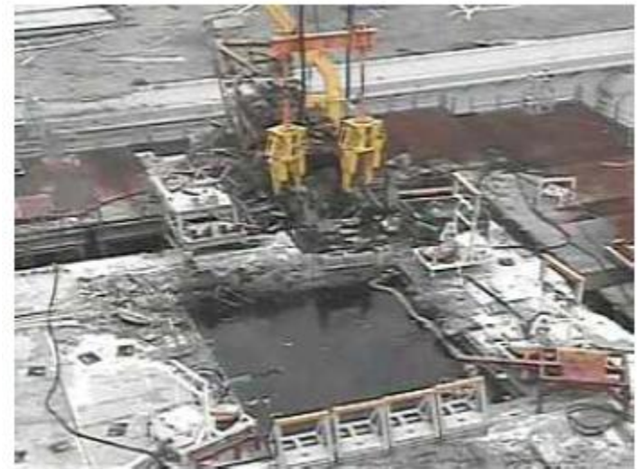
Removal of rubles from SF pool of U-3
