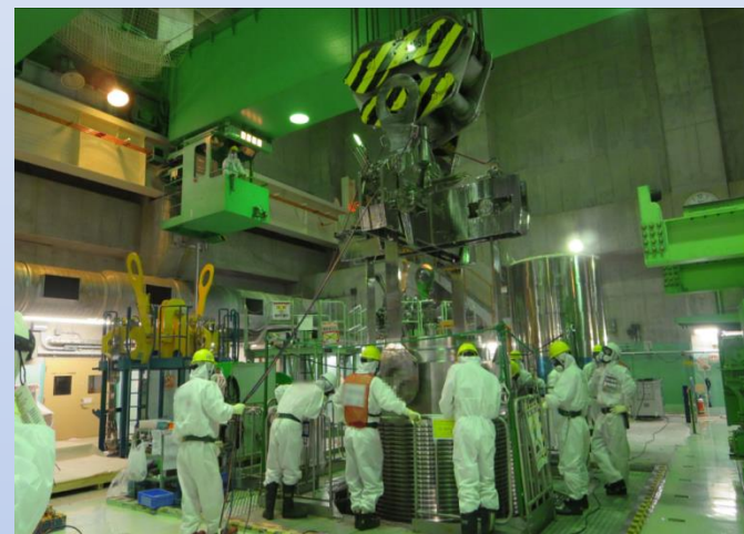
Defueling of the spent fuel pool at Unit 4
