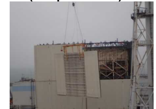
Removal of wall panels (Sep. 2016)
