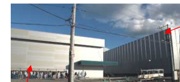
Contractors' office building
