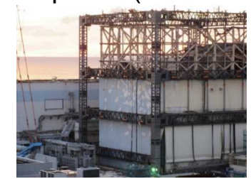
Panels removal completed (Nov. 2016)
