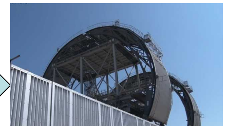
Fuel removal cover (Drill for installment at Onahama)
