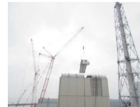
Removal of posts and beams completed (May. 2017)
