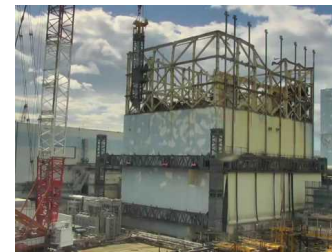
Removal of posts and beams completed (May. 2017)
