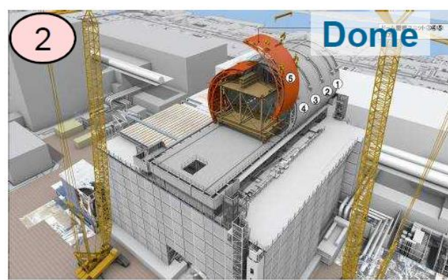
Step of installing Unit 3 fuel removal cover etc.
