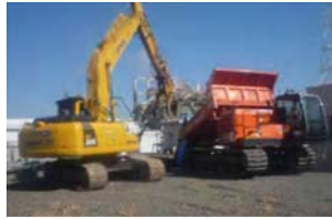
Remotely Controlled Construction Machines
