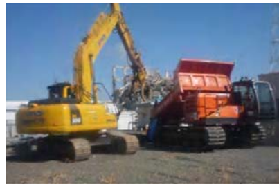
Remotely Controlled Construction Machines
