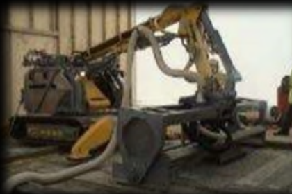
Brokk for Remote Operations Trawsfynydd
