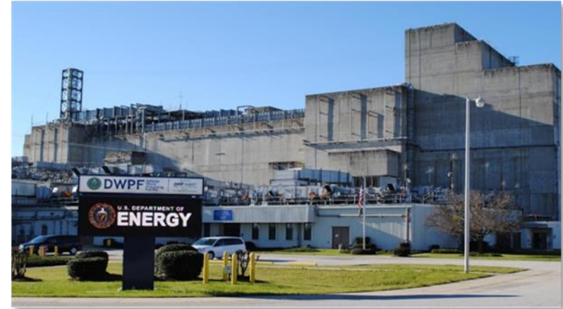
Defense Waste Processing Facility
