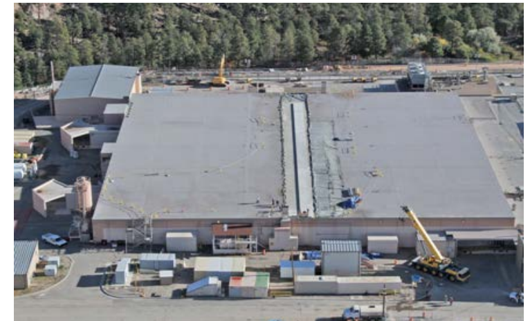
New drag strut at LANL PF-4 for seismic performance
