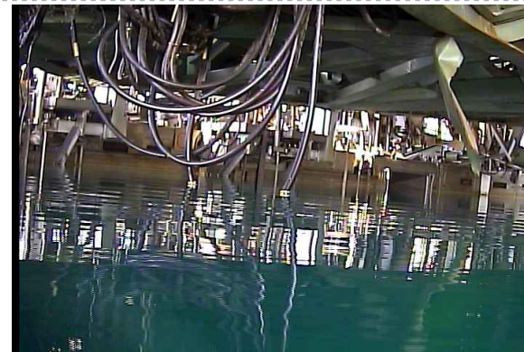
Unit 1 Spent Fuel Pool Photograph taken August 2, 2019
