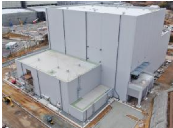
Exterior view of building
